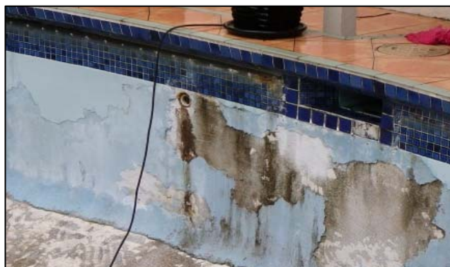
Figure 4 Effects of poor drainage around pool and causing in part delamination of render.
