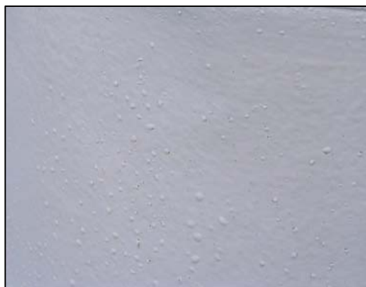
Figure 5 Painted wall showing hydrostatic blisters
