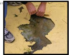
Often some areas of fiberglass will come away easily and others will remain very hard to remove, if at all. Usually it will be necessary to remove the fiberglass where possible and replace OR feather edge the bigger patches leaving clean, bear concrete, fill any remaining holes with epoxy and hope the remainder of the fiberglass that is currently well adhered remains so. Ideally, ALL fiberglass needs to be removed no matter how well adhered.
