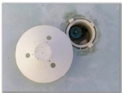
Fig 1: Typical hydrostatic valve assembly
