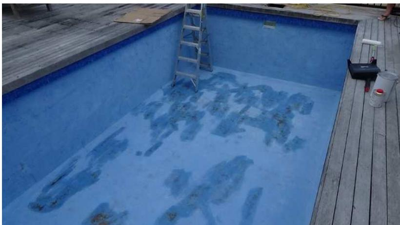
**Prepping the pool using Epotec WB Sealer on the bare concrete areas.**
