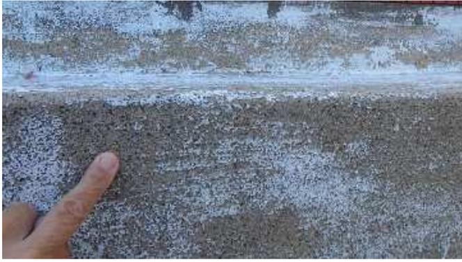
The original surface with bare concrete and Chlorinated Rubber paint.
